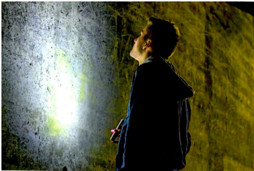
Third Place – Andrew Kotlar Monongahela, PA, Branch 670
